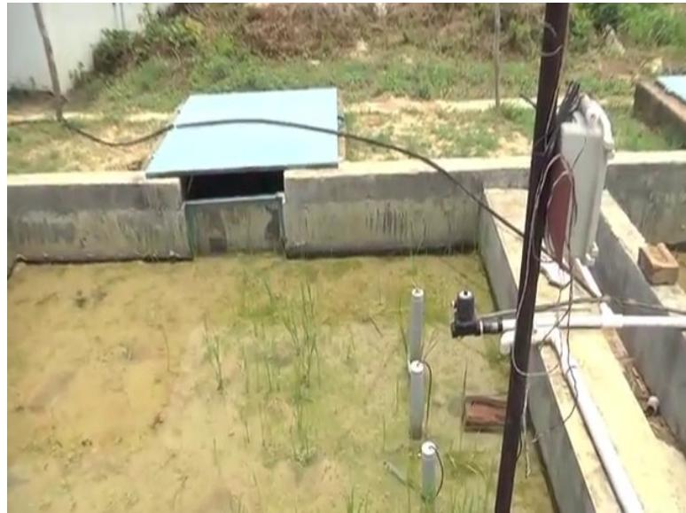
So, what is going to happen is the pump you know it is going to turned on will be turned on and the water is going to be you know the field is going to be irrigated by those this solenoid valves. So, as you can see over here the valve has been turned on just now and the field is going to be irrigated with the water because there is no I am not adequate water in the field.
